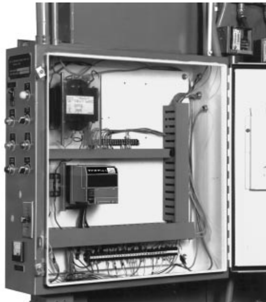
Fig. 9. Electrical panel installation.
